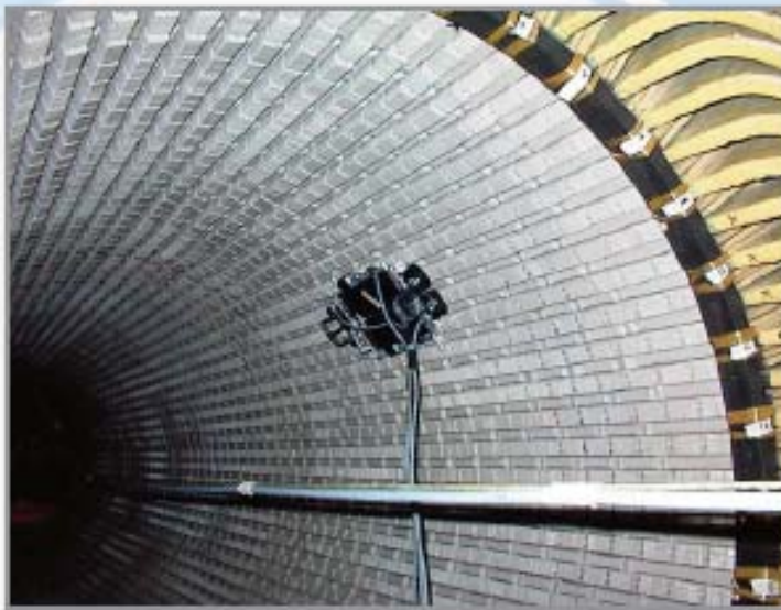
Robotic test in progress (RV feature is optional)
